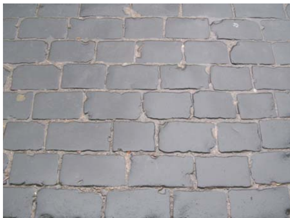
Fig. 23. The pavement from the 1930s made of the Precambrian Volhynian basalt
