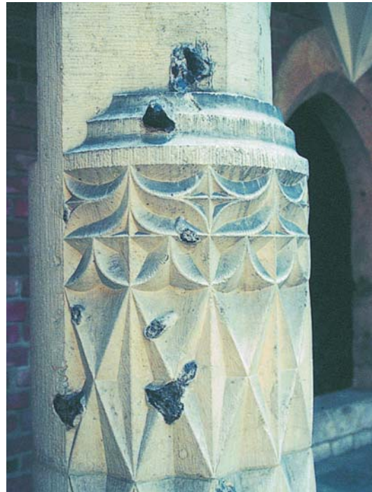
Fig. 12. A bulging flint concretions in a "crystal" column of the Collegium Maius inner courtyard
