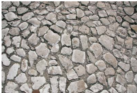
Fig. 1. An old pavement constructed of fragments of the Upper Jurassic limestone; the old, removed pavement of the Main Market square looked the same. All photos by J. Rajchel
