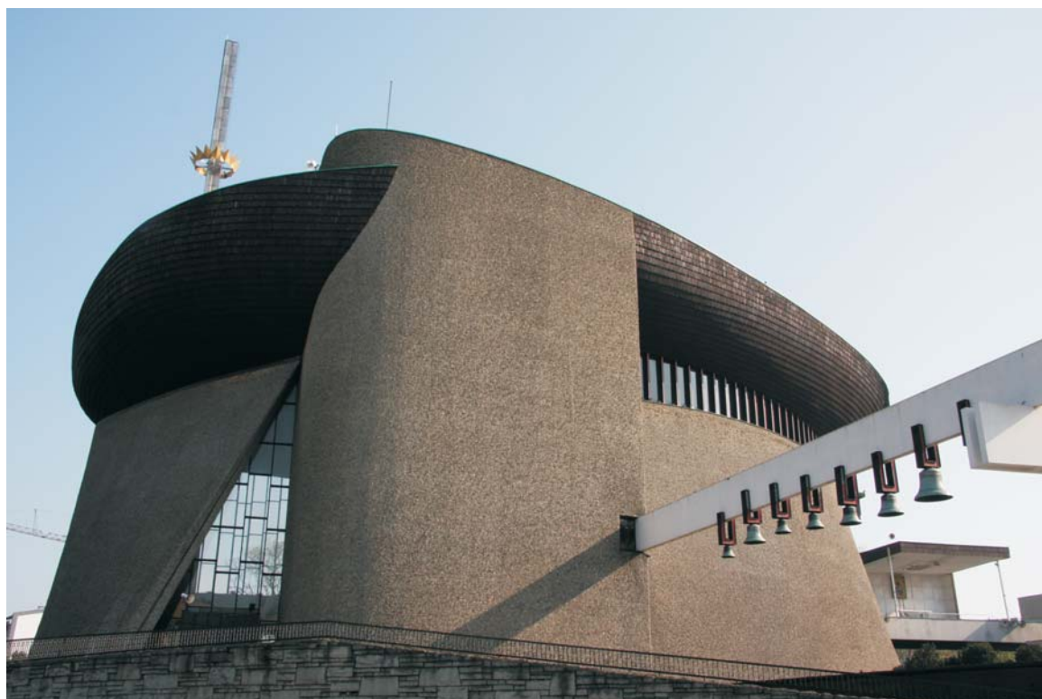
Fig. 20. The Church of the Arc from the 1970s, the first post-war church in Nowa Huta; its walls are lined with pebbles of the Tatra granite
