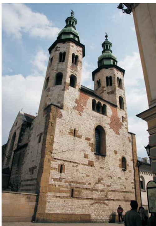
Fig. 2. The Romanesque church of St. Andrew built of limestone blocks ( petit appareil ) and a Carpathian sandstone; the end of the 11 th century
