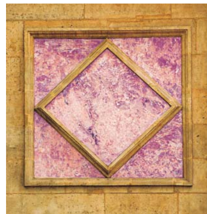
Fig. 9. The decorative element made of the Paczółtowiec limestone in the facade (ca 1630) of the Church of St. Peter and Paul
