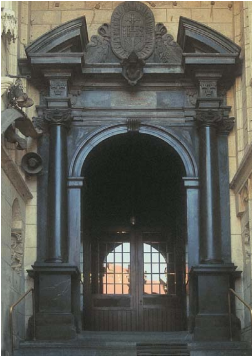
Fig. 4. The Baroque portal from 1636 of the Wawel Cathedral constructed of the black Dębnik limestone
