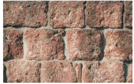
Fig. 11. A fragment of the wall at the Wawel Hill built of the Filipowice tuff
