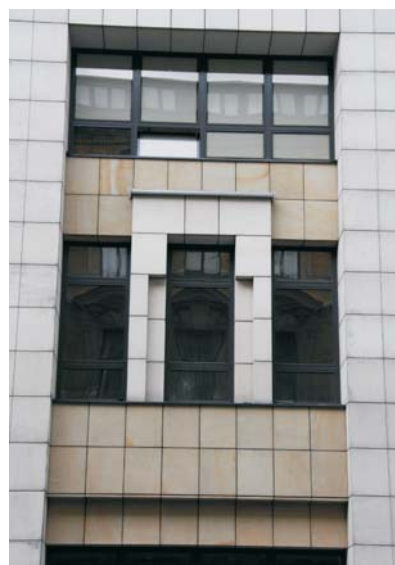
Fig. 19. A fragment of the present-day facade of the building of the Academy of Fine Arts built of the Istebna sandstone (Carpathian Mts) and Jurassic white Szydłowiec sandstone (the margin of the Świętokrzyskie Mts)
