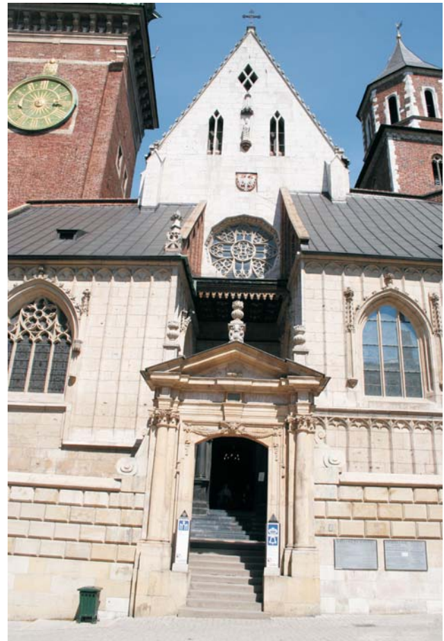
Fig. 6. The Gothic Wawel Cathedral from the 14 th century. The walls built of the Jurassic limestone ashlar ( grand appareil ); the Baroque wall surrounding the cathedral and the gate constructed of the Triassic diplopore dolomite date back to 1619
