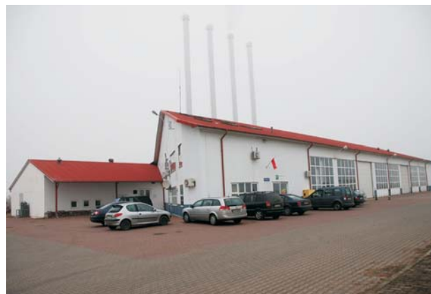
Ryc. 1. Ciepłownia geotermalna w Pyrzycach. Fot. B. Noga Fig. 1. Pyrzyce geothermal heat-generating plant. Photo by B. Noga
