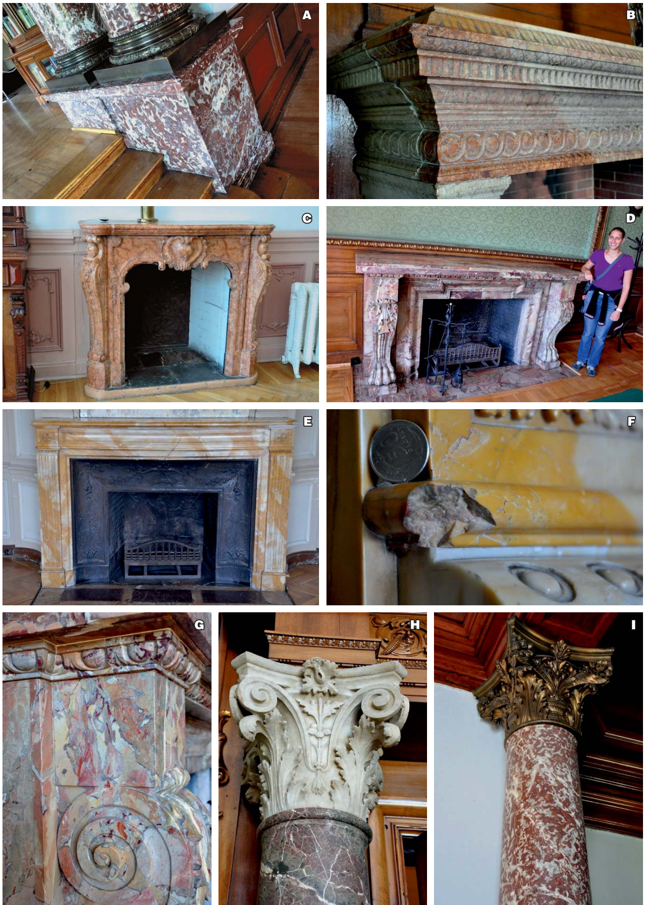
Fig. 7. Moszna Castle – stone decoration of the interiors: A, F – red and white marble columns in the Library; B–G – fire places in representative rooms made of several types of limestones and marbles; H – column of a portal in a representative room, made of purple ophiolite with head in white marble (see text for details)
