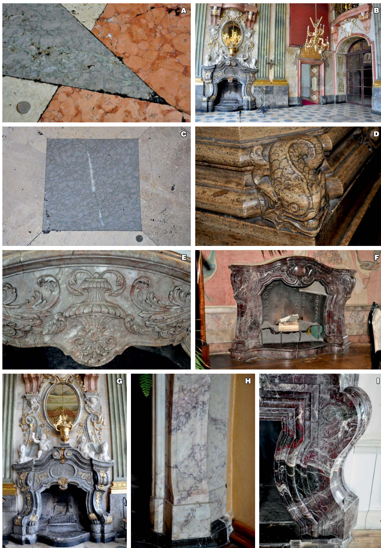
Fig. 4. Książ Castle – stone decoration of the interiors: A–C – examples of “marble” floors; D – column base decoration in the “travertine corner”; E–I – marble fireplaces (see text for details)
