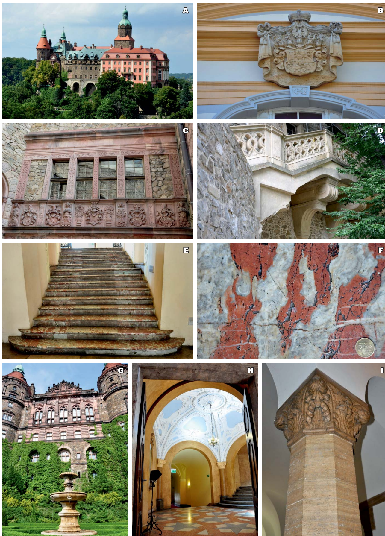
Fig. 3. Książ Castle (A) and examples of usage of local and exotic stones (B–I); B – cartouche of the Hochbergs’ family made of Upper Cretaceous sandstone; C – red sandstone decoration of the internal yard; D – sandstone balustrade of an eternal stairwell; E – stairs made of Rosso di Francia marble; F – Rosso di Francia marble; G – the SW façade decorated with red sandstone; H – corridor paved with Rosso di Verona and grey and light creamy limestones; I – travertine column in the “Travertine Corner” (see text for details)
