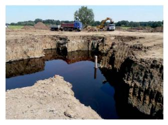
Fig. 11. An example of sanitation in the area surrounding the old re-abandoned wells. Contaminated soils are excavated, contaminated groundwater pumped away. Staré Pole u Nesytu (Propagační materiál PKÚ, 2014)
