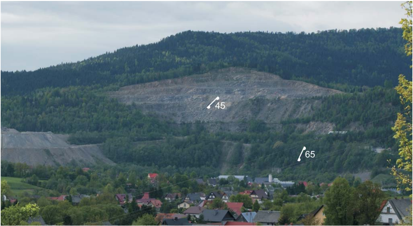
Fig. 7. View of the Osielec quarry with thick-bedded sandstones of the Magura Fm.
