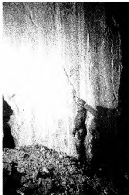
Fig. 3. Exposed fault surface, which facilitated breakdown processes, collapsed debris are visible on passage floor, Żyrafiowy Passage
