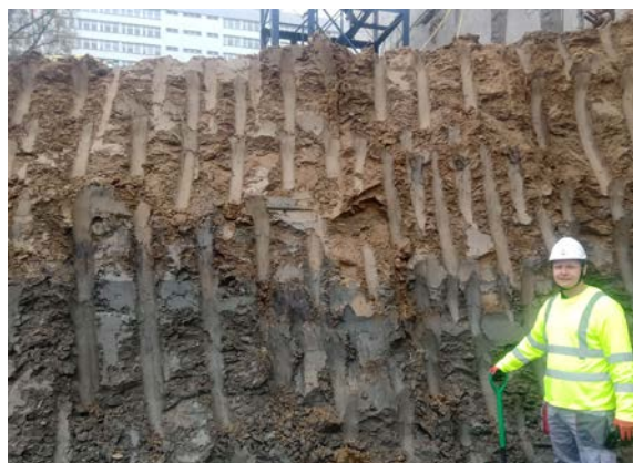
Text-fig. 3. Two glacial till horizons (upper – brown and lower – grey) in a foundation excavation at the Ochota Campus of the University of Warsaw (photo by P. Zawrzykraj).
