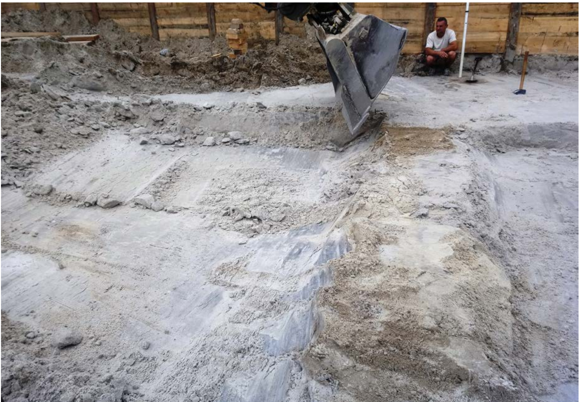
Text-fig. 6. Unnatural grey colour of cemented fluvial sand (originally yellow in colour) forming blocks and crumbs during mining. Picture taken at point c4 (as located in Text-fig. 1).
